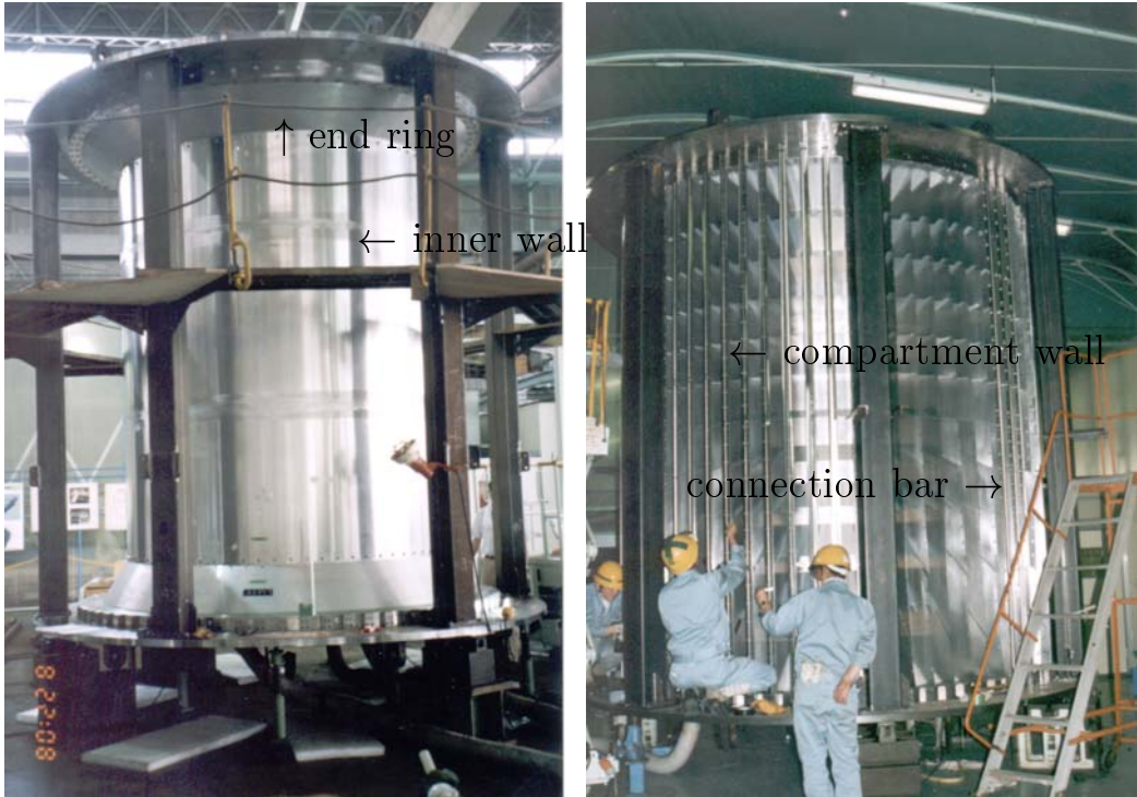
Figure 4.20: Mechanical structure for holding the \text{CsI(Tl)} counters. (Left) Before and (Right) after attaching the compartment wall to the inner wall.
